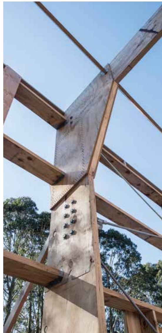
LVL supplied directly from the Marsden Point Mill to the fabricator, Carters manufacturing.
