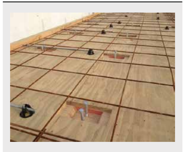
Photo 5: TCC Floor with Mesh Installed
