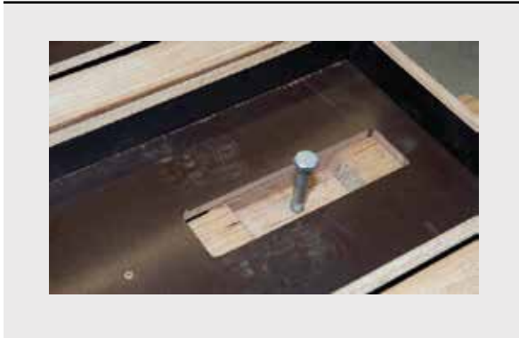
Photo 1: Fabricated Trapezoidal Notch
