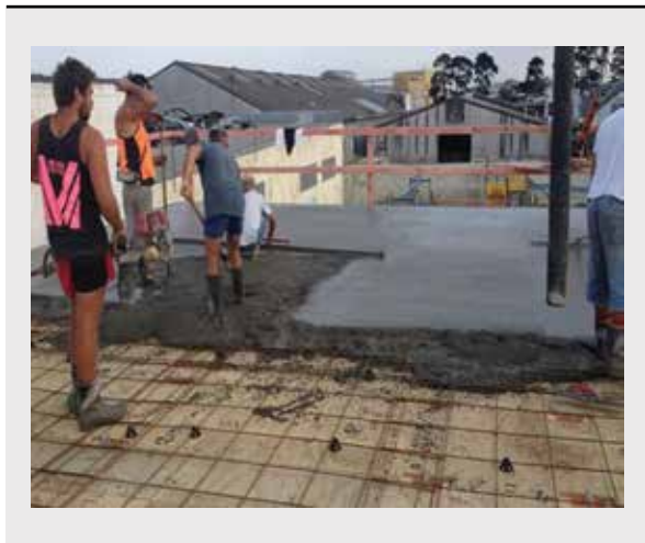
Photo 6: TCC Floor Laying Concrete Slab
