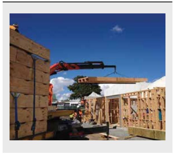
Photo 3: TCC Floor Delivery & Installation
