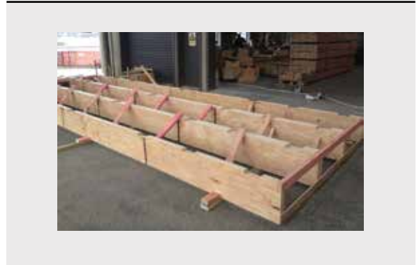
Photo 2: Fabricated Section (ex. Plywood Formface)
