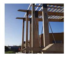
The 12 m vertical height accommodates the hanger doors that provide an opening of 28 m by 9 m and required some careful thought, said Lisa. "We had to design the end wall to fit the doors and the top support. Probably deflection was the hardest thing to work around.
