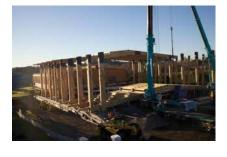
By adding some veneer at 90 degrees to the typical grain of Futurebuild LVL you give the individual piece of timber more stability." The flexibility of Futurebuild LVL in size and type allowed Holmes to create Futurebuild LVL based box beams to clear span this large open area.
