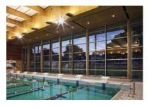
Graham Upton of Upton Architects preferred the more slender look of the Futurebuild LVL beams. "We didn't want a chunky looking roof structure so once we told our engineer we wanted to pursue a timber structure he was keen to use the new technology with hySPAN."
